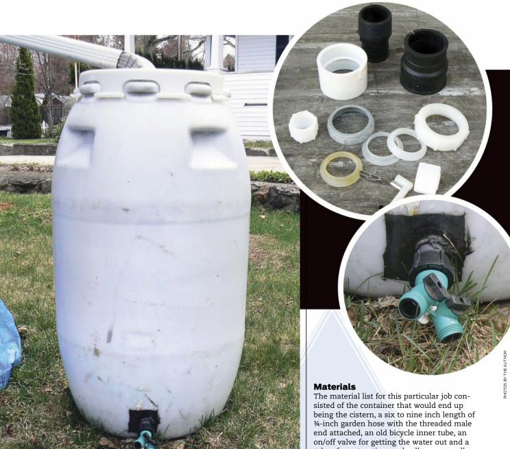
My design was very simple. When it rains the water comes off my roof and is caught by metal gutters which then transfer the water to the ground and away from the house. To make the cistern work I would simply tap into the gutter and allow the water to run into the container. All I needed to do is to figure out a way to access the water from the cistern, without removing the cover, to water my garden. I went ahead, drew up my plans and gathered the materials for the project.
